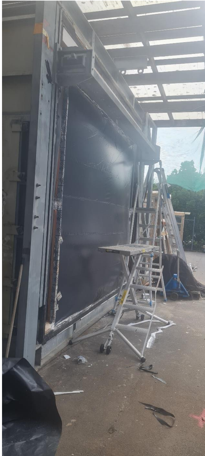
Figure 31: Airtightness testing with sample sealed.
