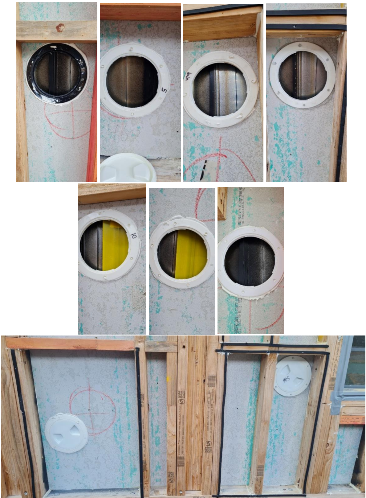
Figure 37: 'Port-holes' in rigid wall underlay to allow access and pressure manipulation
