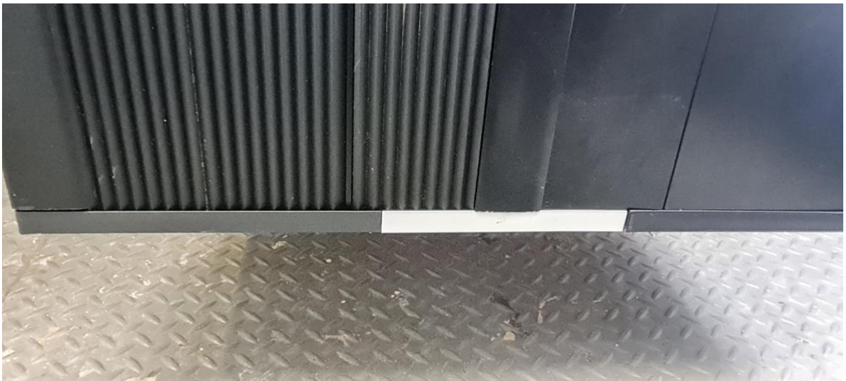
Figure 26: Cladding vertical joint between profiles and footer
