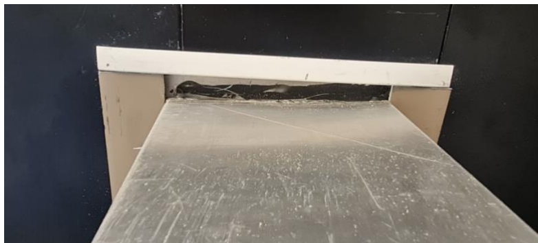
Figure 27: Parapet saddle flashing
