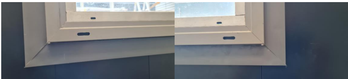
Figure 24: Window drainage
