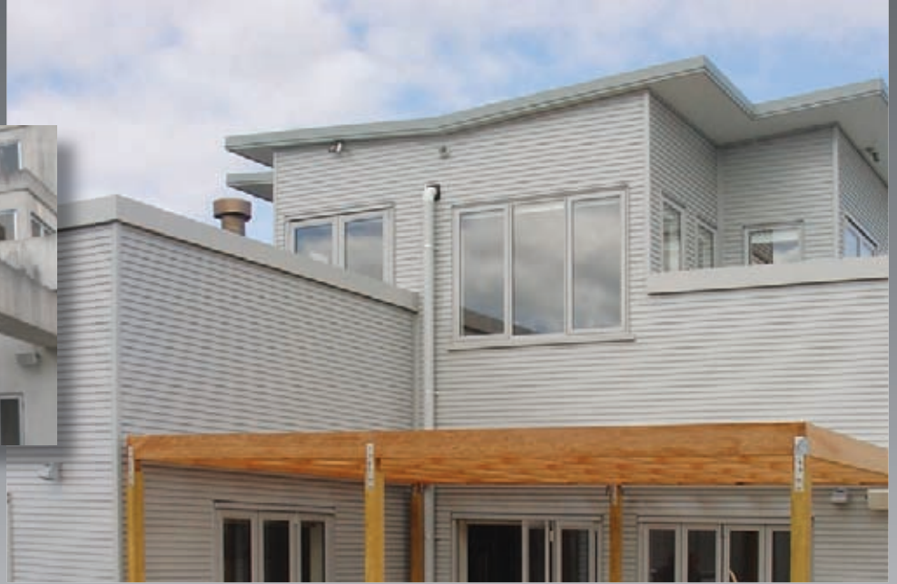
After re-clad with Louvre 60 - Horizontal
